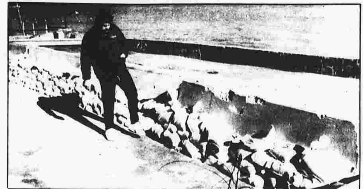
Boistering sea walls
